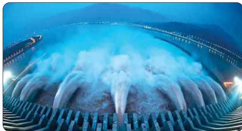
Proposed Inga project to meet bulk of power needs for SADC region
