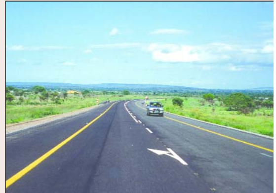
The N4 toll road links Maputo and Witbank.
