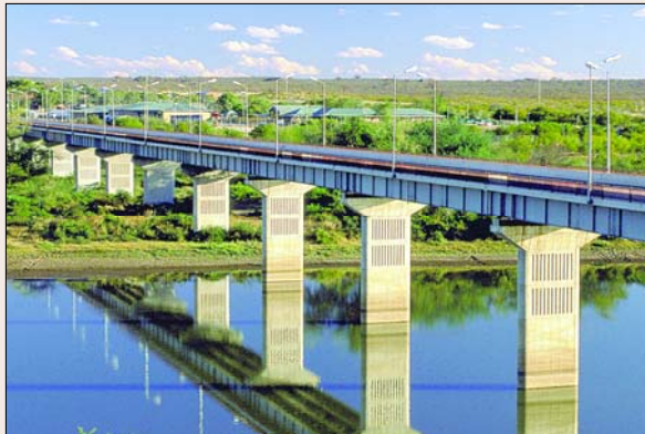
Bridge infrastructure such as this one over the Limpopo river facilitates movement of people across the region.
