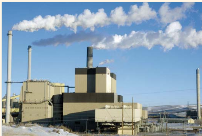
Emissions such as this one from a cement factory in South Africa are harmful to the environment.
