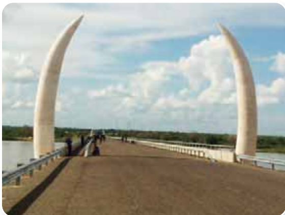
The opening of the Unity Bridge over the Ruvuma River between northern Mozambique and southern Tanzania in May 2010 marked another milestone towards deeper regional integration. The bridge means that the two countries, separated by a river but with longstanding historical and family ties, can further strengthen their political, social, economic and cultural relations, and expand intra-regional trade.
