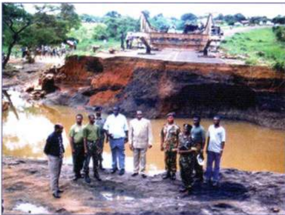
Restoring a bridge on Malawi's M1 road
